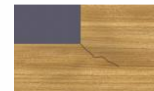
NO CLAIM WILL BE ENTERTAINED FOR CRACKING ARISING OUT OF GROOVE CURRYING OR L-SHAPE
